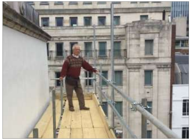
Fig. 4. The author on the scaffolding.
