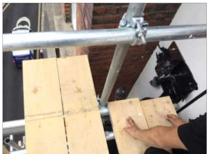
Fig. 5. October 2021: working on the installation of the gnomon.
